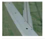
I-Beam to Rim bolted connection is strong and provides a clean surface for the sheeting and its clamping
