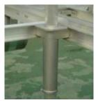
Landing leg sleeves are keyed into the I-Beam frame
